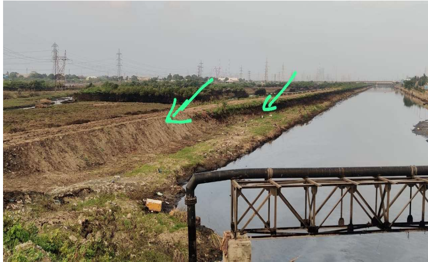
Figure 13: B canal possibly breached and oil stain covered.
