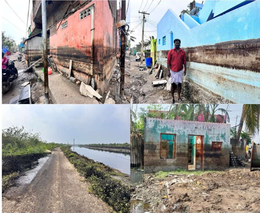
Figure 6: Oil marks observed in the residential localities of Ernavoor.
